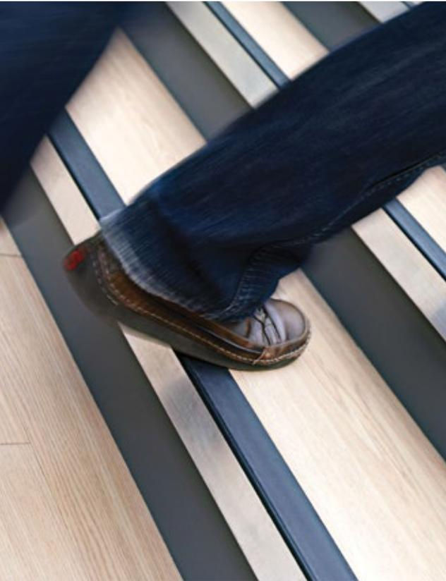
Stair edgings, or stair nosings as they are also referred to, should be used to highlight the edges of steps in public and commercial buildings, in line with Approved Documents M (ADM) and K (ADK) of The Building Regulations 2010 and BS 8300:2009+A1:2010, which look at the design of buildings and their ability to meet the requirements of less able people.
